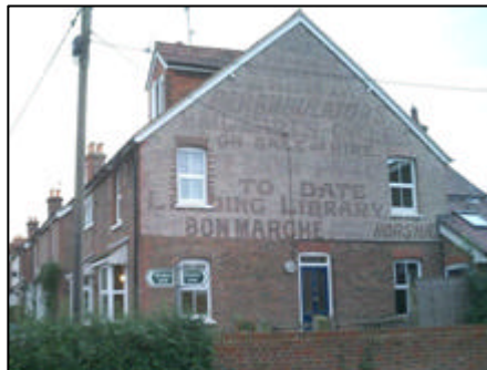
Hayes Lane Downs Link Crossing
